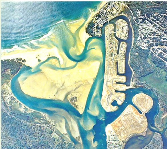
May 1978, during construction of Noosa Sound Canal Estate
