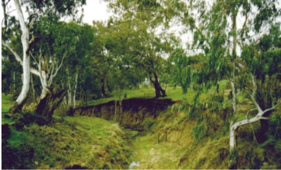
Gully erosion along a creek in Bathurst, NSW.
