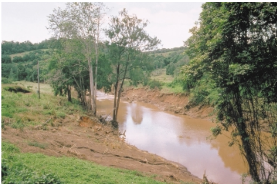
Unstable stream banks resulting from clearing of riparian vegetation contributes to river silt loads.
