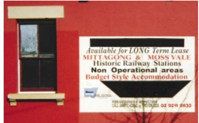
Surplus Mittagong (NSW) Railway Station building being offered for lease for alternative use.
