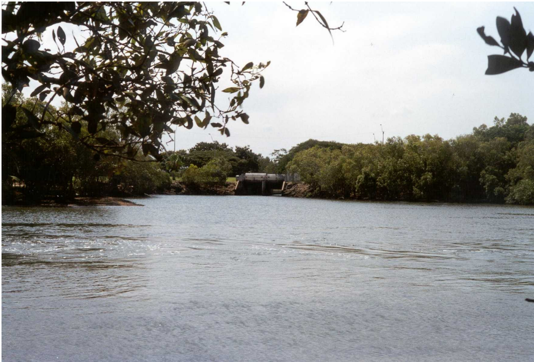
Figure 1. (Site 1) The Ross Creek just below the tidal gates (in the background) at the junction with the Woolcock Street stormwater drain
